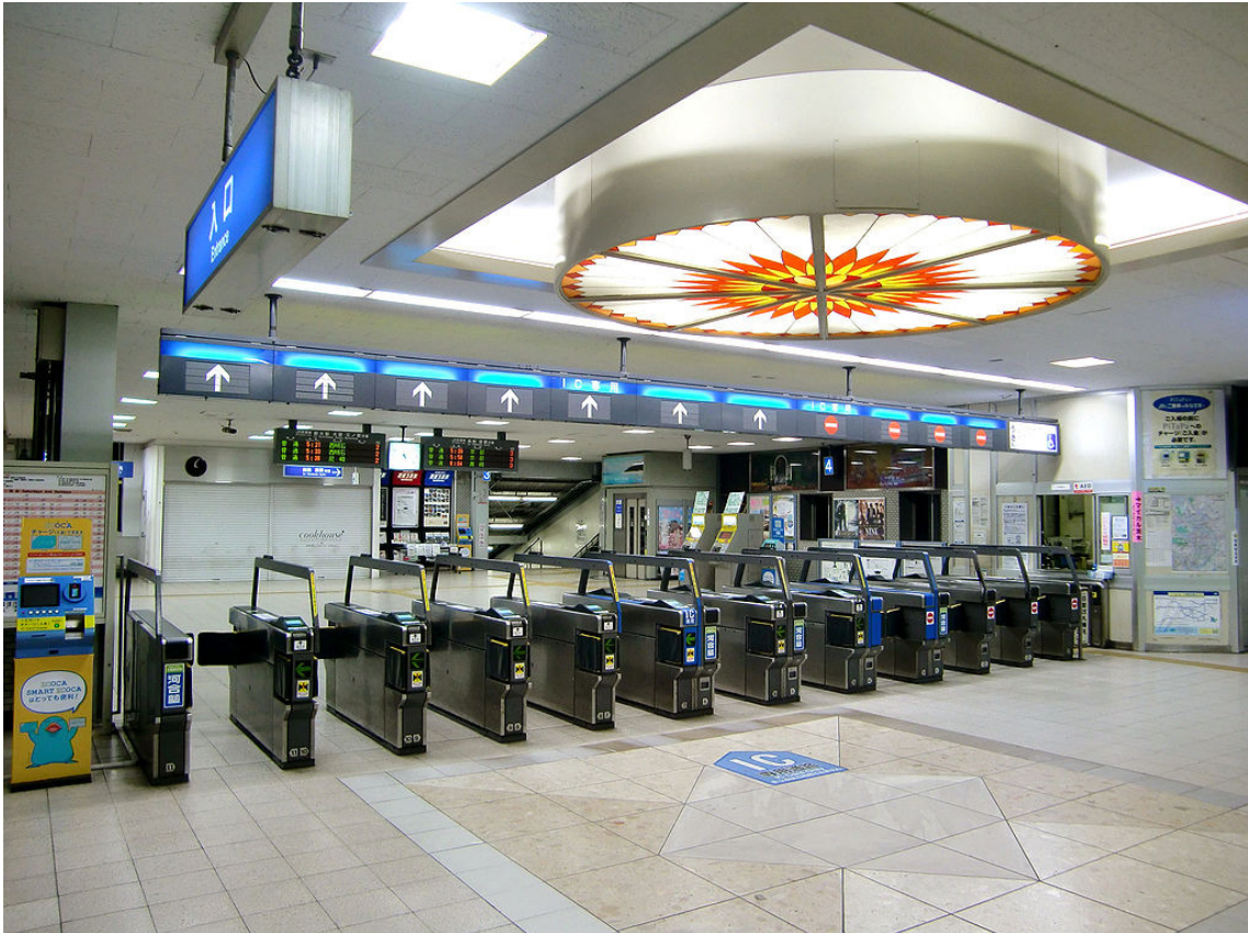
A wicket with automated devices (JR Ibaraki Station, Osaka)
